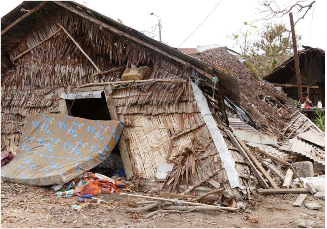
Cyclone Pam made downfall on Vanuatu (2015), destroying and damaging 15,000 homes (Source: Silke von Brockhausen/UNDP Vanuatu)
